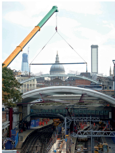
Thameslink programme, Farringdon Station redevelopment achieved an ‘Excellent (90%)’ rated CEEQUAL award.
